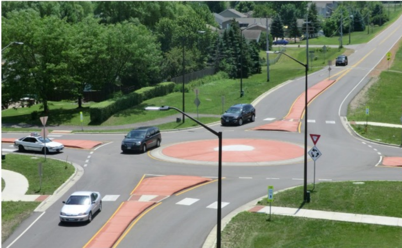
Example of a single-lane roundabout. Source: FHWA
